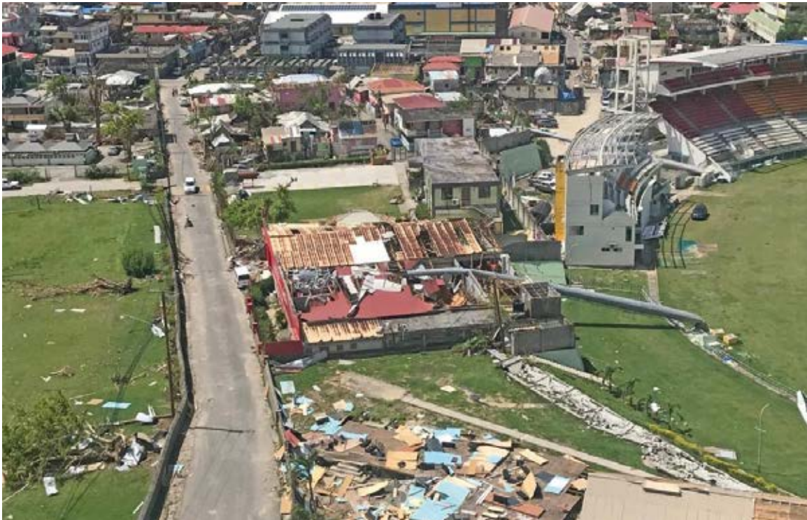
Roseau, the capital of Dominica, after Hurricane Maria in 2017.
